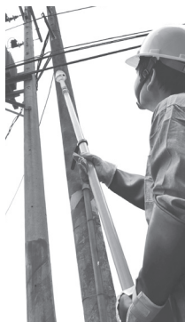
Fig. 3: Voltage detection for overhead lines
